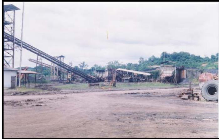
Foto 4. Instalasi pengolahan batubara (crushing, screening)
